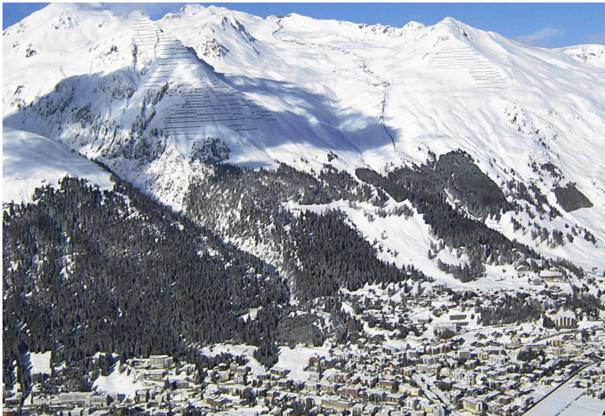
Improved protection against natural hazards, including avalanches, through intentional afforestation, adapted forest management (densification) and additional technical measures in Parsenn (Switzerland) between 1945 and 2007
