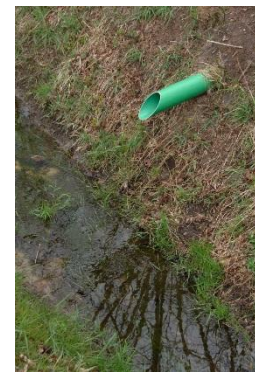
Figuur 4: Grondwaterlozing (RIONED)
